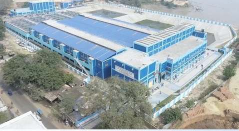
250MLD WTP Project, Uttarpara, West Bengal, Completed (VaTech Wabag)
