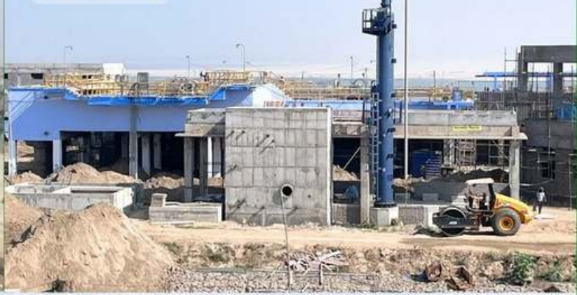
100MLD STP Project, Patna, Bihar in progress (VaTech Wabag)
